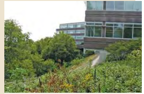
Development abutting the bluff must not encroach on the steep-wooded slopes.
