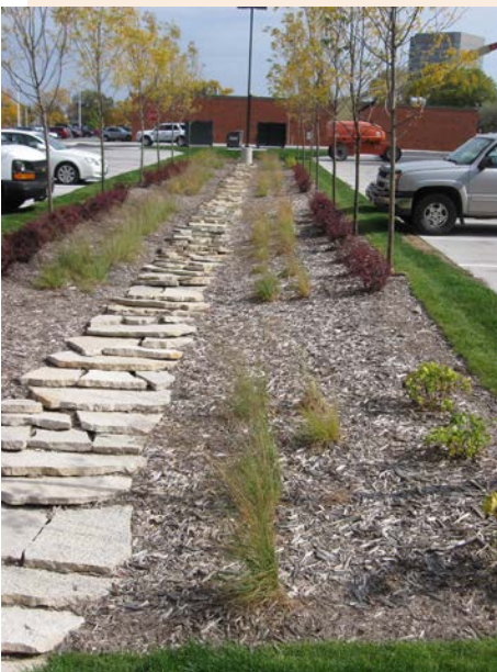
Rain water garden in parking lot
