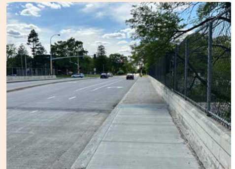
Looking west along E 86th Street bridge, showing the sidewalk edge abutting the street
