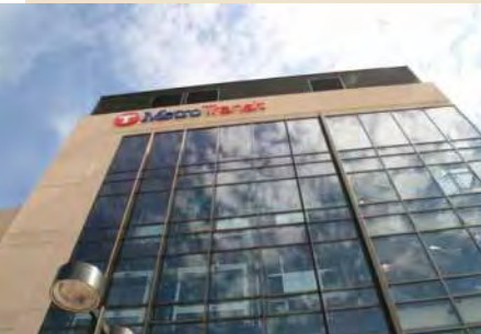
The 28th Avenue Park and Ride is served by LRT and several bus routes.
