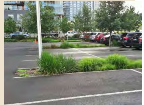
Bioswales within a parking lot help collect and filter runoff.
