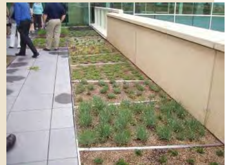
Planted “green roofs” increase the amount of pervious surface on a development site.
