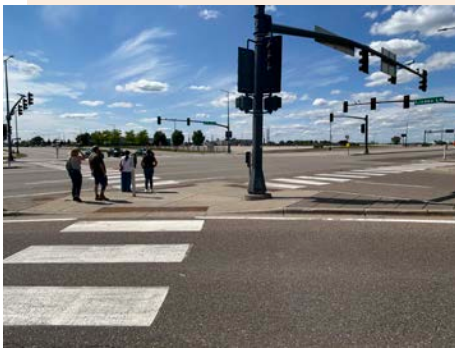
Free right turn lane looking northwest from the corner of the quasi-public space by the AC Marriott Hotel
