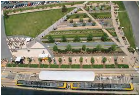
Central Station Park combines plaza space with open green areas that can accommodate larger gatherings.
