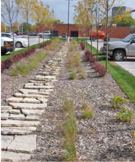
A rain garden/infiltration trench demonstrates sustainable stormwater management.
