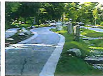
STORMWATER SWALE ADJACENT TO PATH
