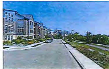
ROADWAY ADJACENT TO THE UPPER LANDING
