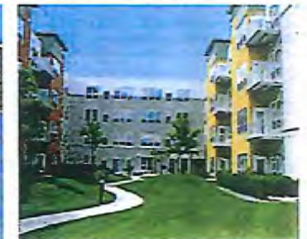
PATHWAY BETWEEN BUILDINGS
