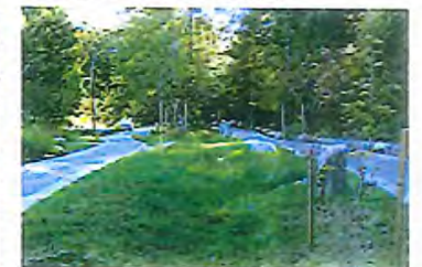
STORMWATER SWALE BETWEEN PATHS
